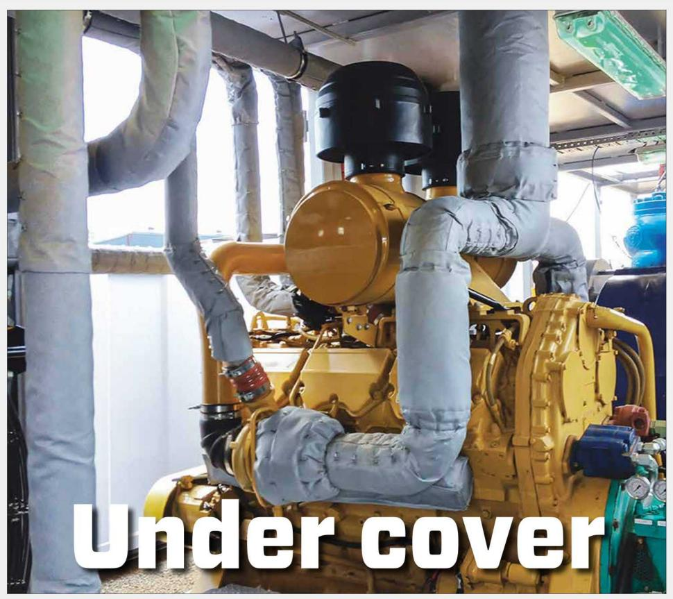
Pyrotek's thermal insulation blankets were custom-made to suit the exhaust manifolds, turbocharger and turbocharger air outlet plumbing to completely wrap any heat sources in this installation.
