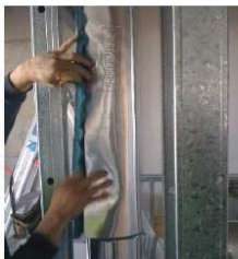
Wrap each segment with an overlap
