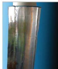
Tape along the longitudinal overlapped length
