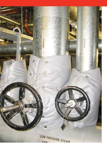
Pyrotek speciality products custom makes and designs covers that utilise our range of fabrics, felts and blankets to suit a variety of conditions from cryogenic to high temperature metal smelting. There is an increasing demand for removable insulation covers for all types of high temperature equipment. Our covers provide excellent personal protection from heat and are easy to remove and replace when performing maintenance.
