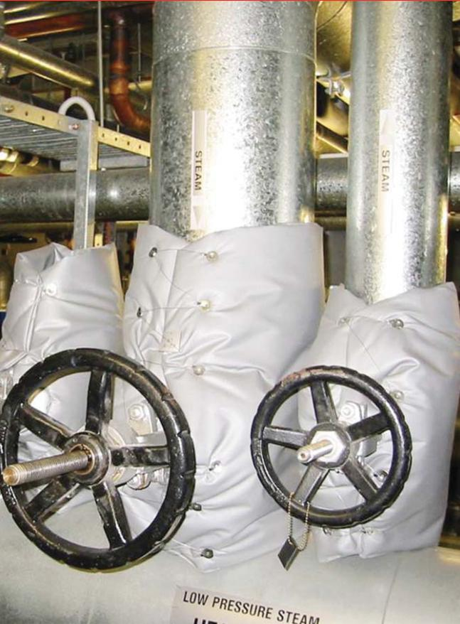
Pyrotek speciality products custom makes and designs covers that utilise our range of fabrics, felts and blankets to suit a variety of conditions from cryogenic to high temperature metal smelting. There is an increasing demand for removable insulation covers for all types of high temperature equipment. Our covers provide excellent personal protection from heat and are easy to remove and replace when performing maintenance.
