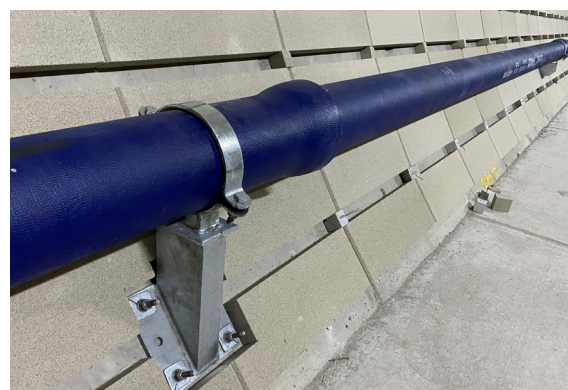
Tunnel application - Reapor installed on the wall
