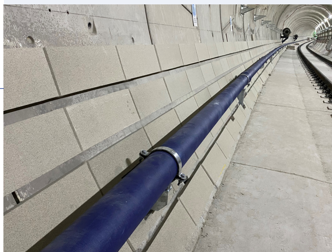
Reapor 625 x 208 panels installed in tunnel application
