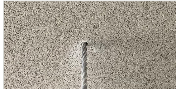
Drill into the centre of Reapor
