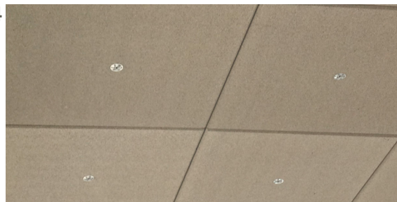
Completed overhead installation
