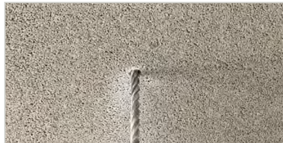
Drill into the centre of Reapor
