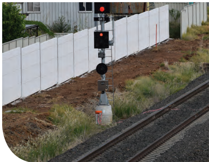
Reapor installed on Noise Wall 1 to protect the Gunnedah community
