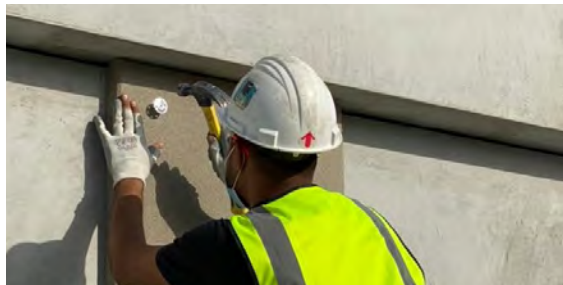
Gently hammer the pin in place
