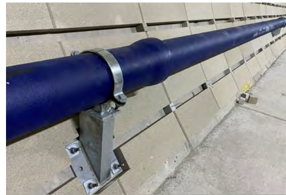
Tunnel application - Reapor installed on the wall
