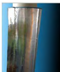
Tape along the longitudinal overlapped length
